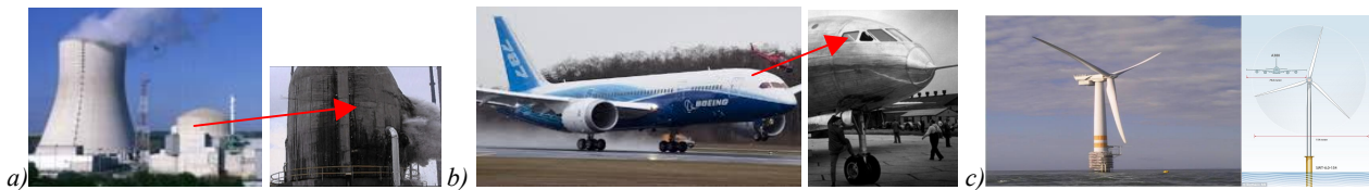
Figure 1. Integrity and durability of (costly) massive composite structures: a) nuclear power plant both existing PWR and new EPR systems - stringent requirement on waterproof containment structure of CBFR composites; b) (European answer to) Boeing 787 Dreamliner, the most fuel-efficient aircraft built of CFRP composites – new requirement on no-return-to-hub for crack reparation; c) large offshore wind-turbine with CFRP composites blades and deep-sea CBRF composites support – requirement of durability and integrity to guarantee operational capabilities under extreme weather conditions for the largest possible offshore turbine blades (larger than A380 wings span).
