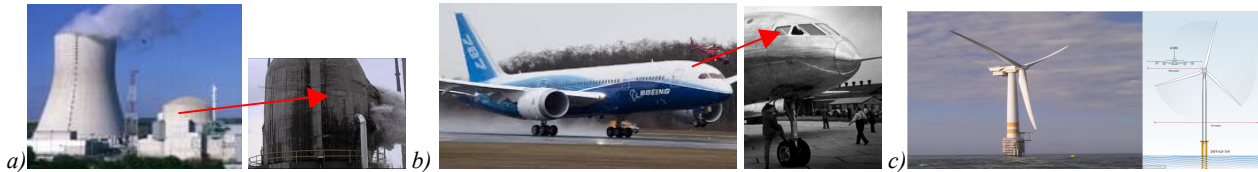
Figure 1. Integrity and durability of (costly) massive composite structures: a) nuclear power plant both existing PWR and new EPR systems - stringent requirement on waterproof containment structure of CBFRC composites; b) (European answer to) Boeing 787 Dreamliner, the most fuel-efficient aircraft built of CFRP composites – new requirement on no-return-to-hub for crack reparation; c) large offshore wind-turbine with CFRP composites blades and deep-sea CBFRC composites support – requirement of durability and integrity to guarantee operational capabilities under extreme weather conditions for the largest possible offshore turbine blades (larger than A380 wings span).
